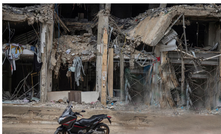
Israel's air raids cause heavy damage to Lebanon.
